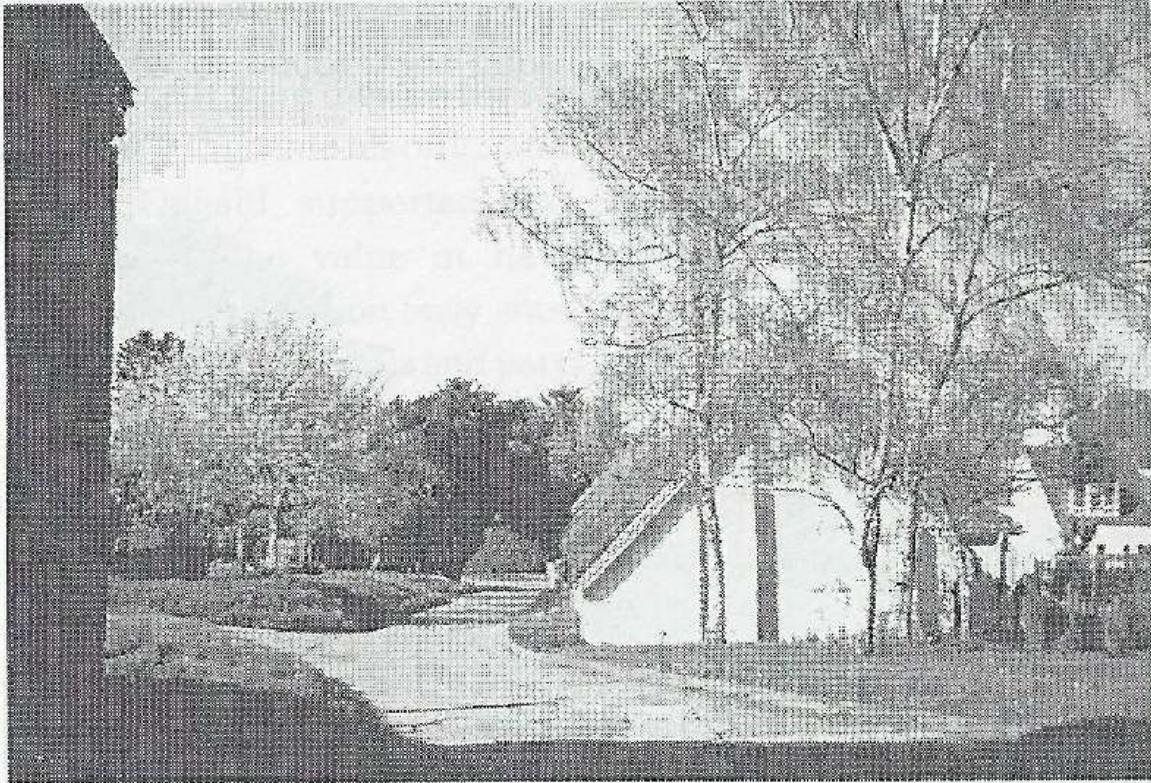
Beyond the Canteen Area looking North
