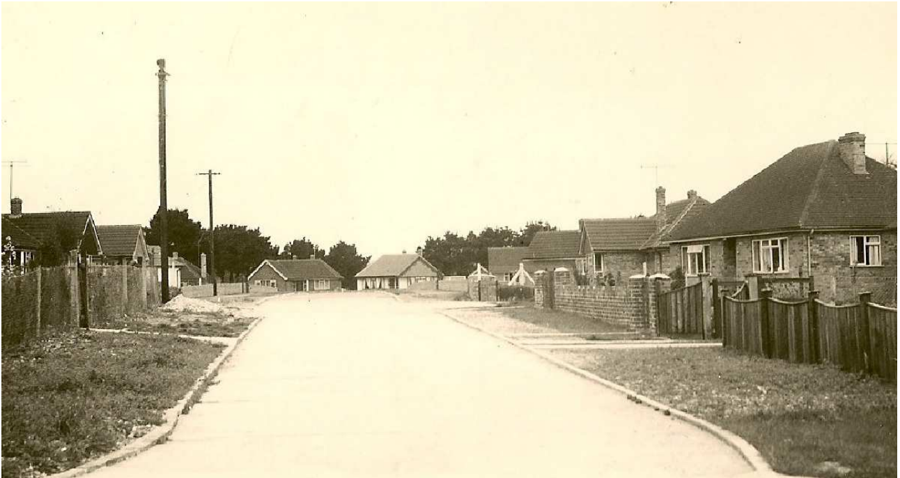
Orchard Close, shortly after construction
